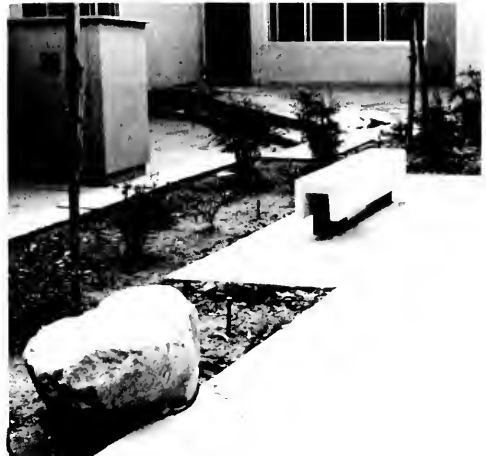
Photo 9. Van Gogh Street Elementary School. Diagonal crack in slab near rock; damage in the concrete steps beyond.
